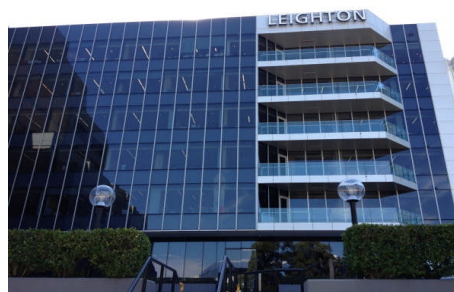
The southern side of the multi storey Leighton Building.
