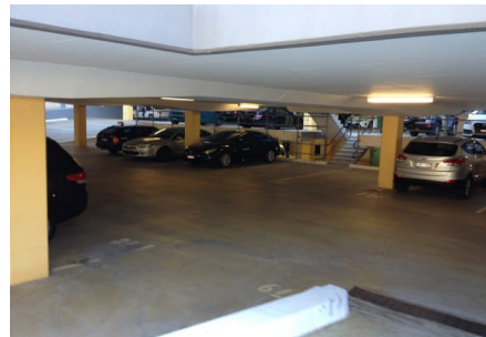
The basement carpark at No.472 with concrete sealed surface in good condition.
